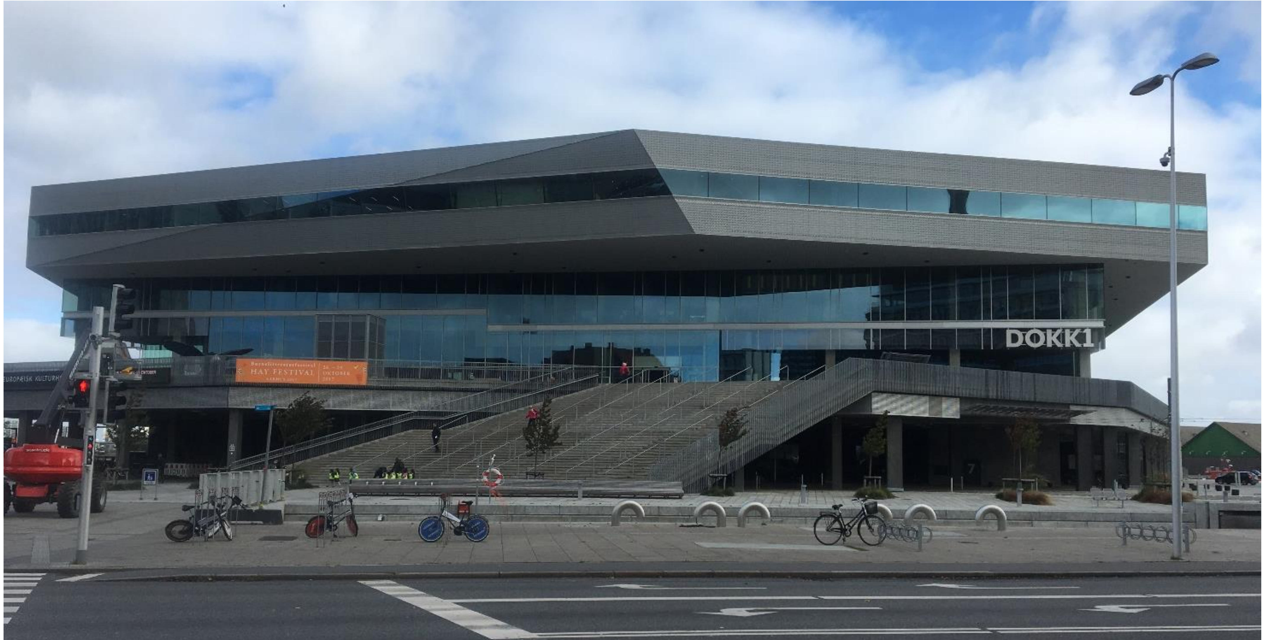
Dokk1, Aarhus, Denmark
